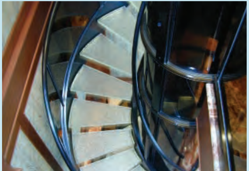
Textured and patterned glass products are being used increasingly for stairs and flooring.
